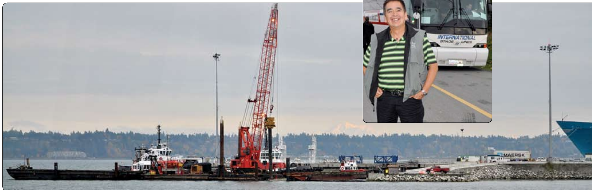
TFN/Matcon joint venture were working on a barge ramp removal.
