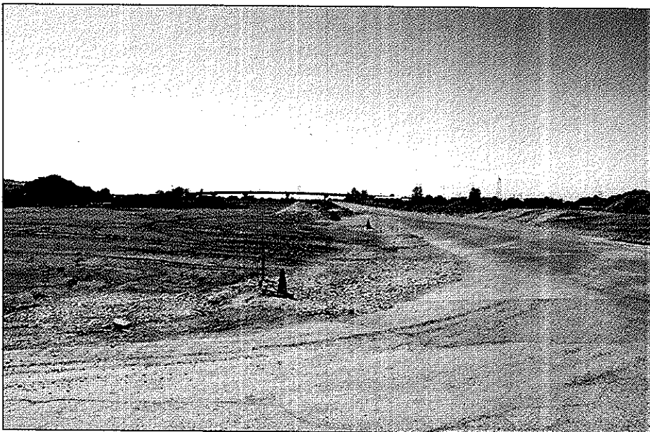
Open opportunity: TFN Economic Development Corp. is seeking partners keen to develop logistics space on this 100-acre tract of land near the Deltaport container terminal
