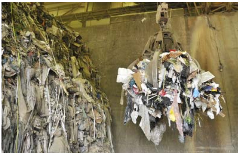
Waste is hoisted by crane into Metro Vancouver's existing waste-to-energy plant in Burnaby.
